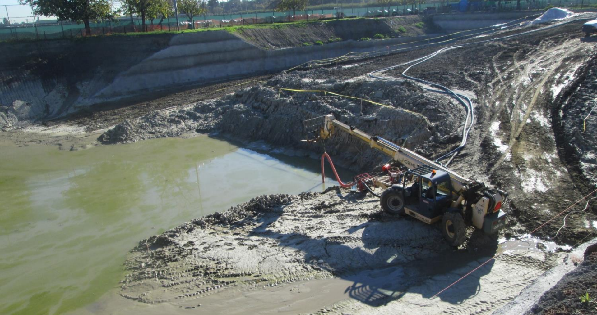
Dewatering after rain storms
