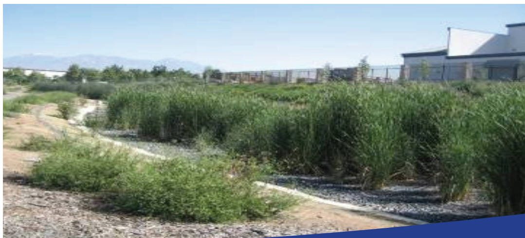
Subsurface Flow Wetlands at Chino Creek Park
