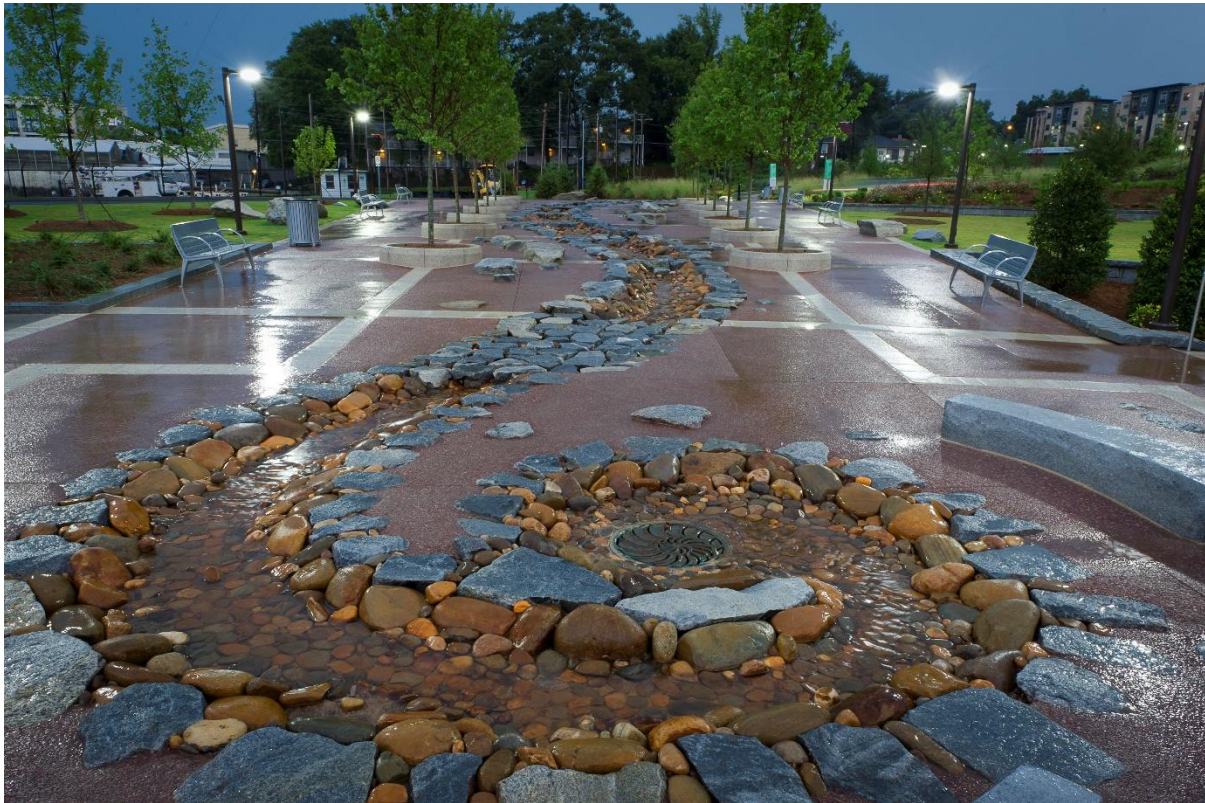
Figure 4. Throughout the park, drainage features are disguised as artistic sculptural elements. This ephemeral channel is lined with river stone and granite to represent Clear Creek, which flowed through the site nearly 100 years ago.
