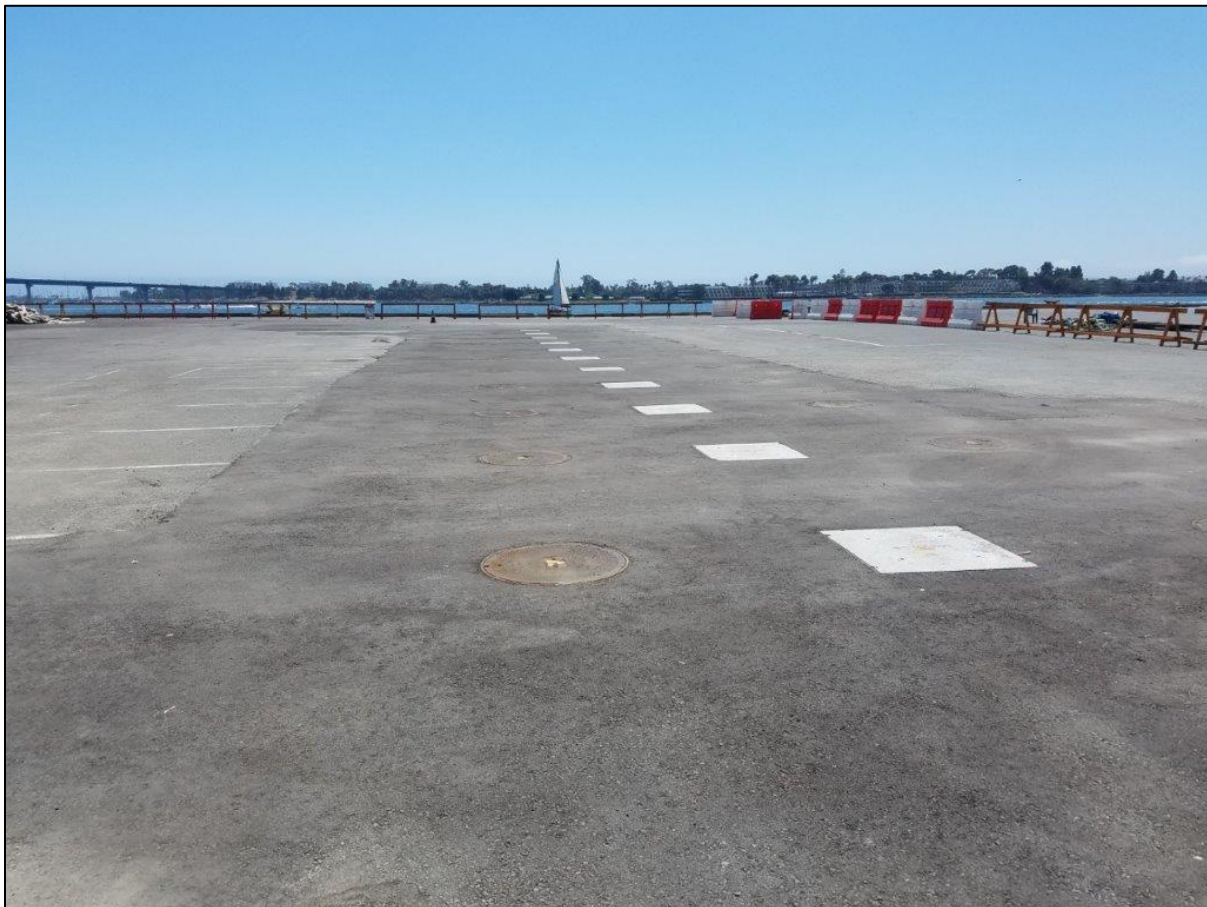
Figure 6. Installed biofiltration units in place with finished pavement
