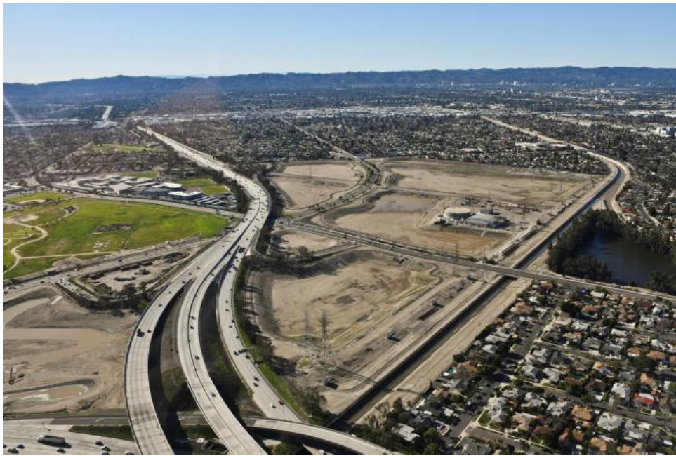
Figure 5. Tujunga Spreading Grounds after Phase 1- Basin Enhancements
