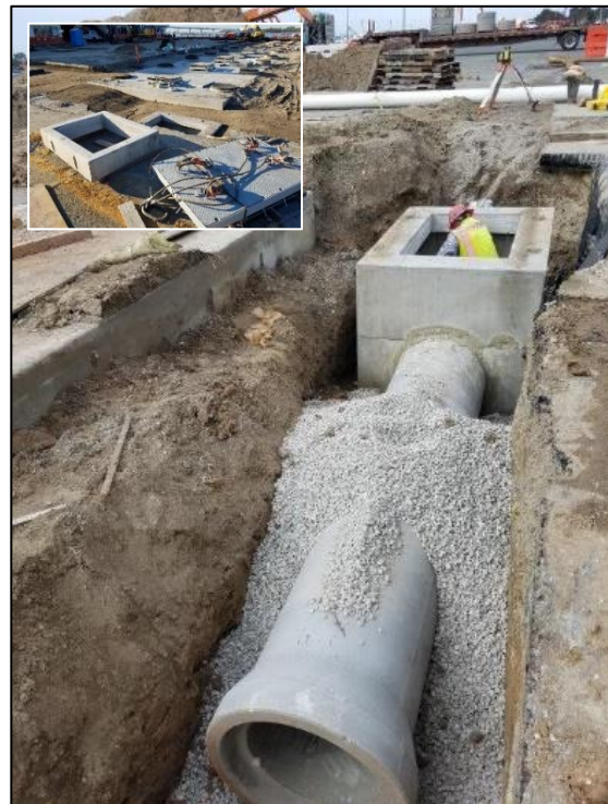
Figure 5. Rocking and grouting of hydrodynamic separator (see inset)
