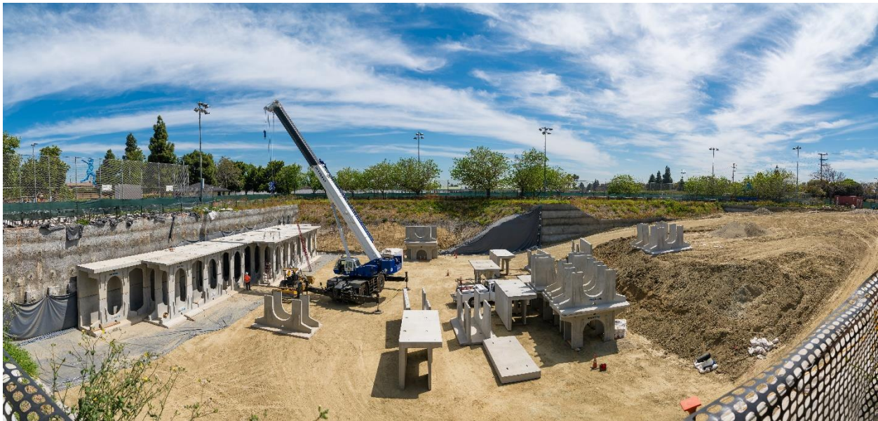
Figure 1: Installation of subsurface stormwater storage chambers (facing east)
