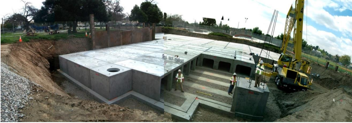
Figure 1: Infiltration Galleries at City's Garvanza Park
