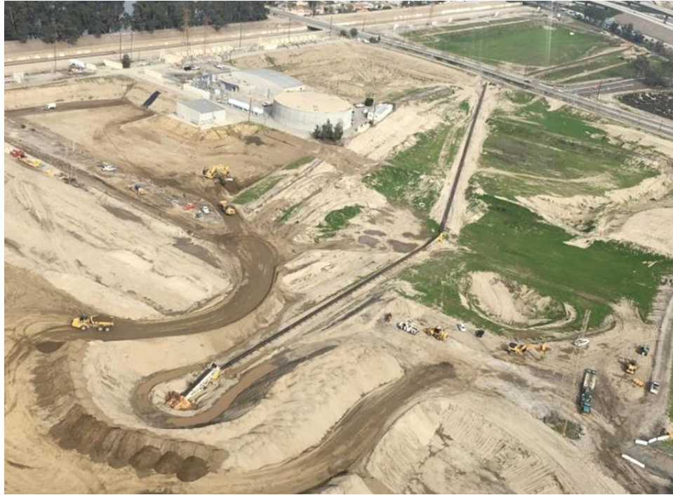
Figure 4. Aerial view of the conveyor belt and the excavation in progress
