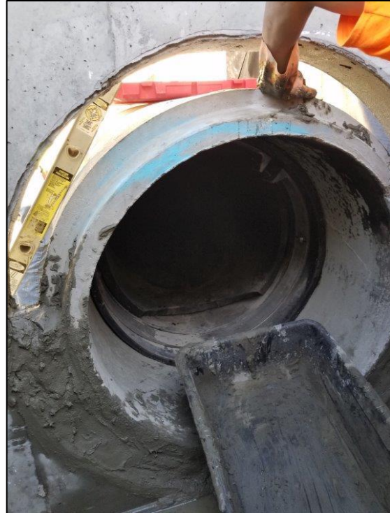
Figure 3. Downstream side of tide gate
