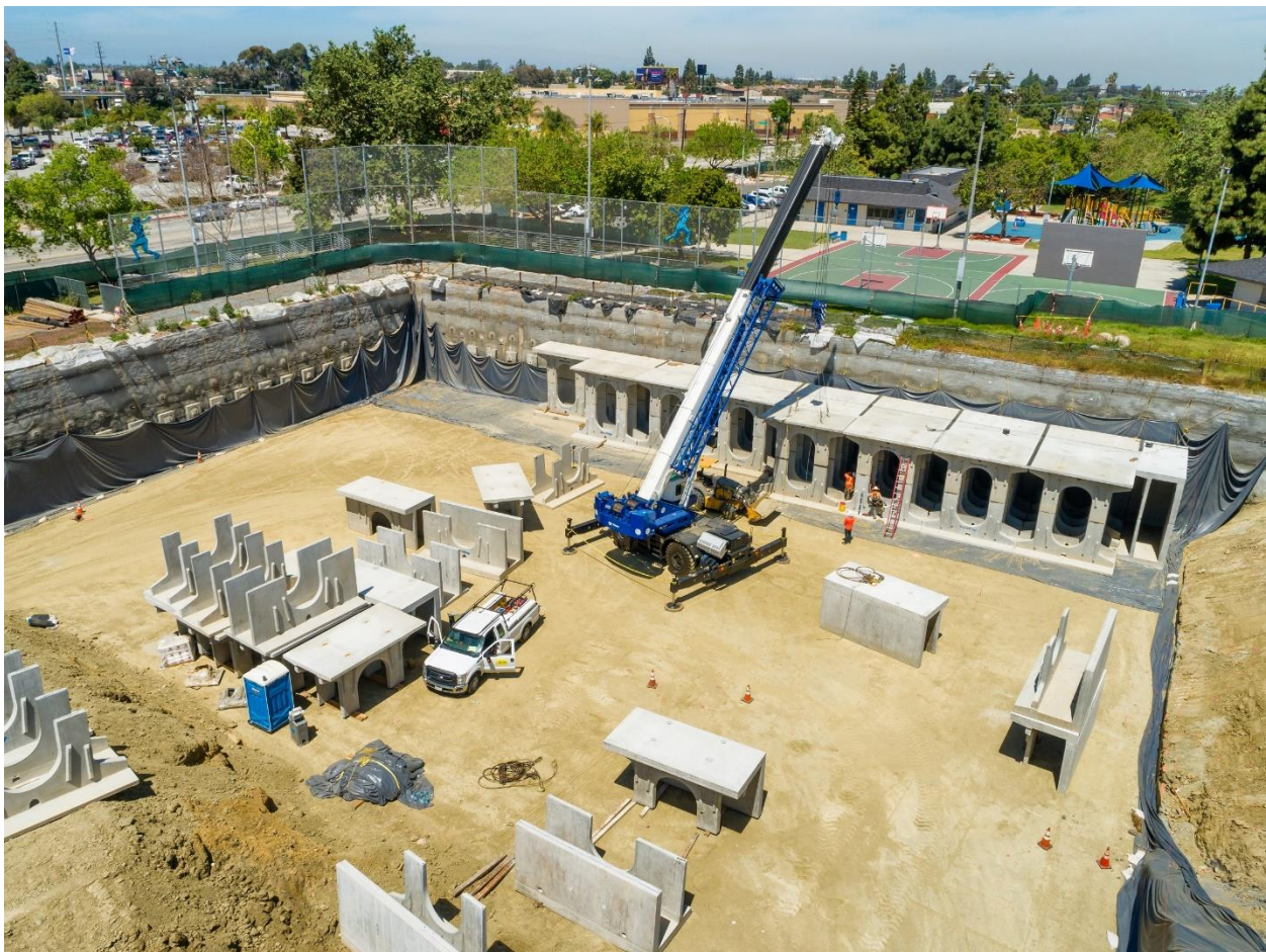
Figure 2: Installation of subsurface stormwater storage chambers (facing north)
