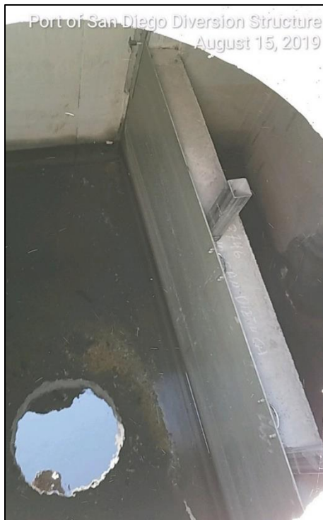
Figure 4. Diversion weir structure
