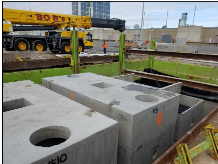
Figure 1. Setting biofiltration units in place
